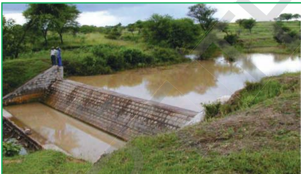
fig-1: Communitybased masonry dam
